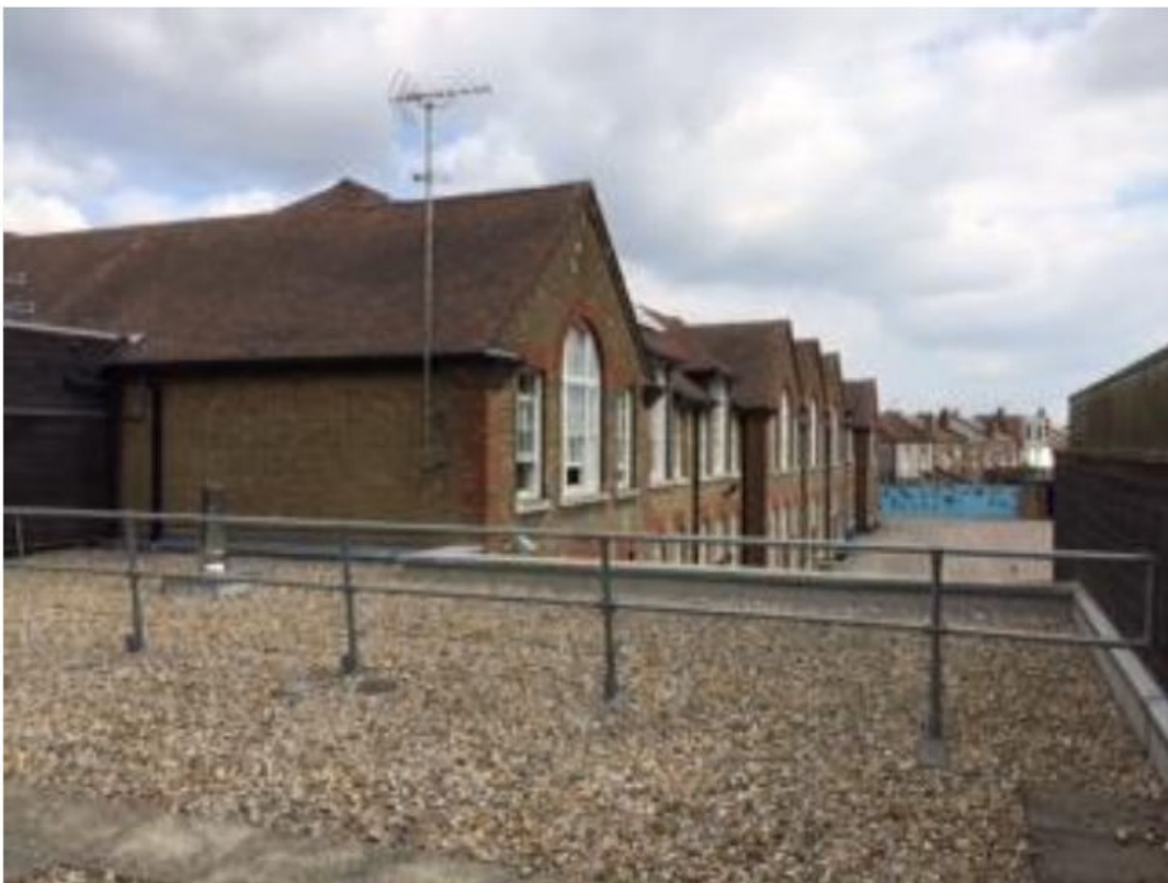
Extension location looking East
