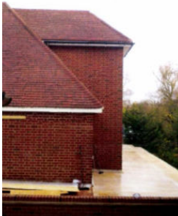
Part of side elevation seen from No 20
