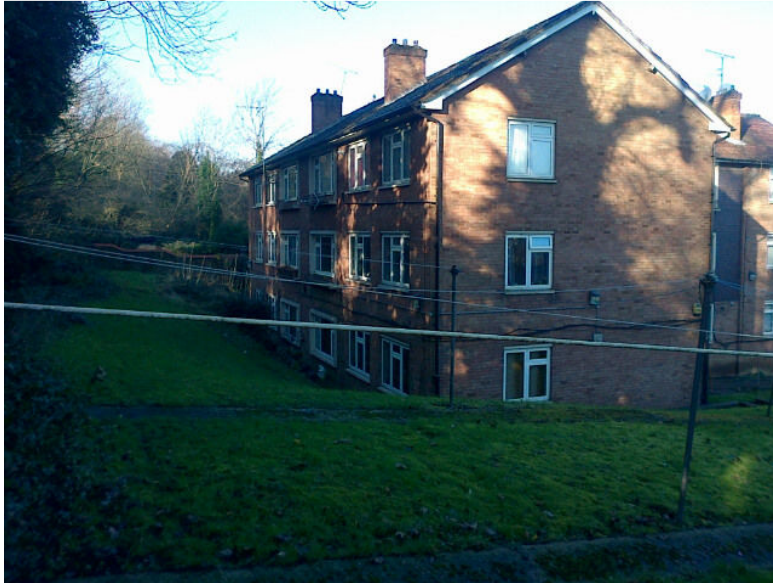
Existing block of flats
