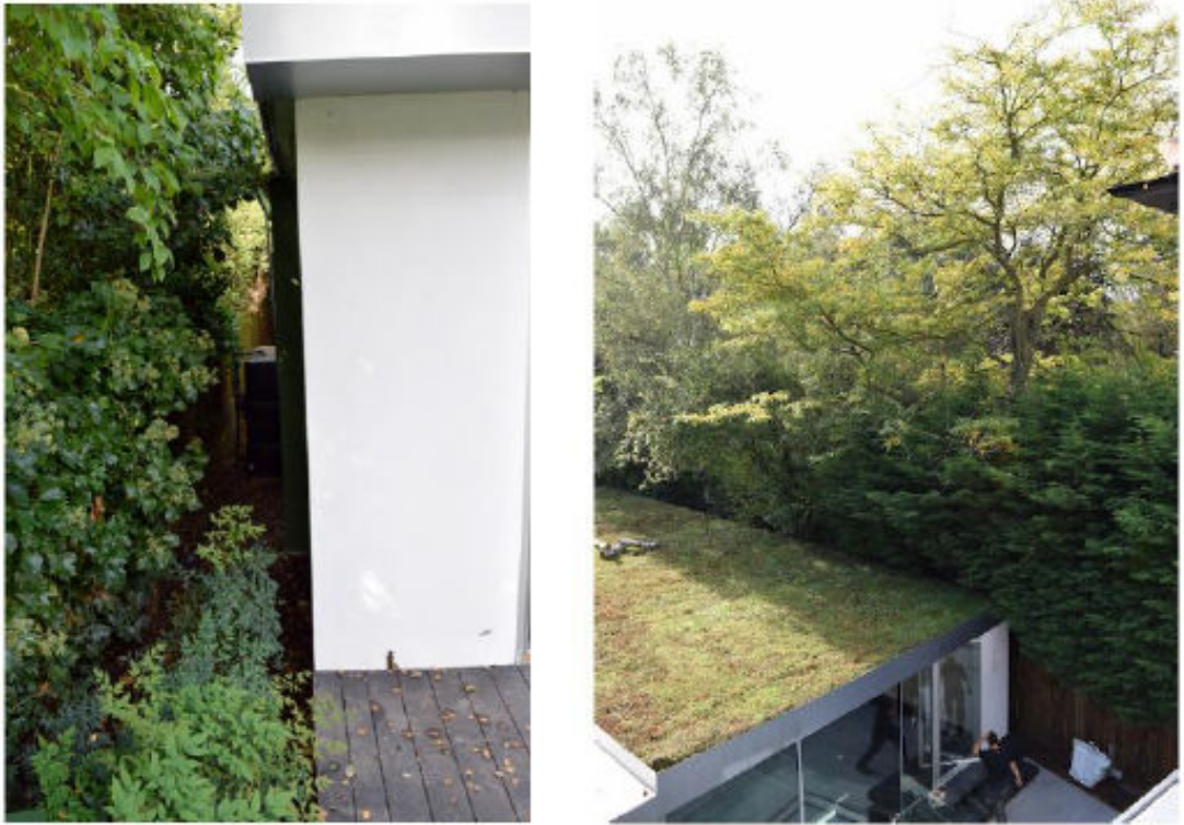
Side/ Roof of Pool House
